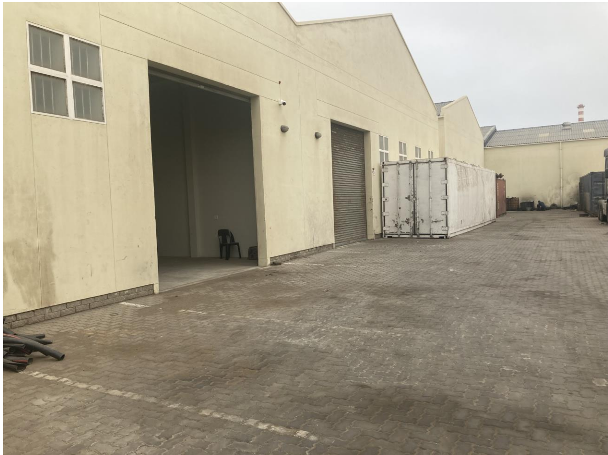
Figure 5: Proposed outdoor flame cutting area of Kontinental Industrial Products (Pty) Ltd., Erf 4616, Light Industrial Area, Walvis Bay (Source: Author).
