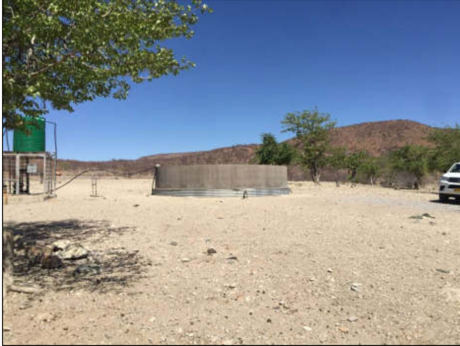
Figure 15: Existing man-made water dam within the EPL area
