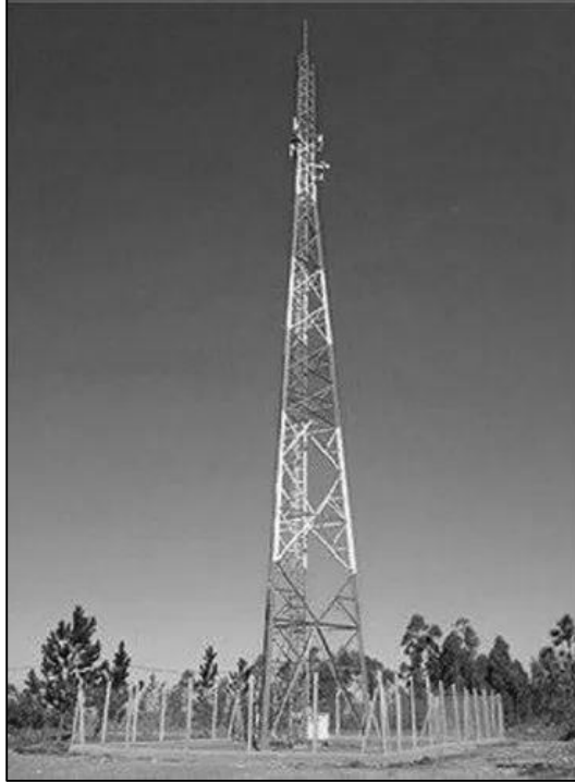
Figure 2: A typical red and white painted lattice tower structure
