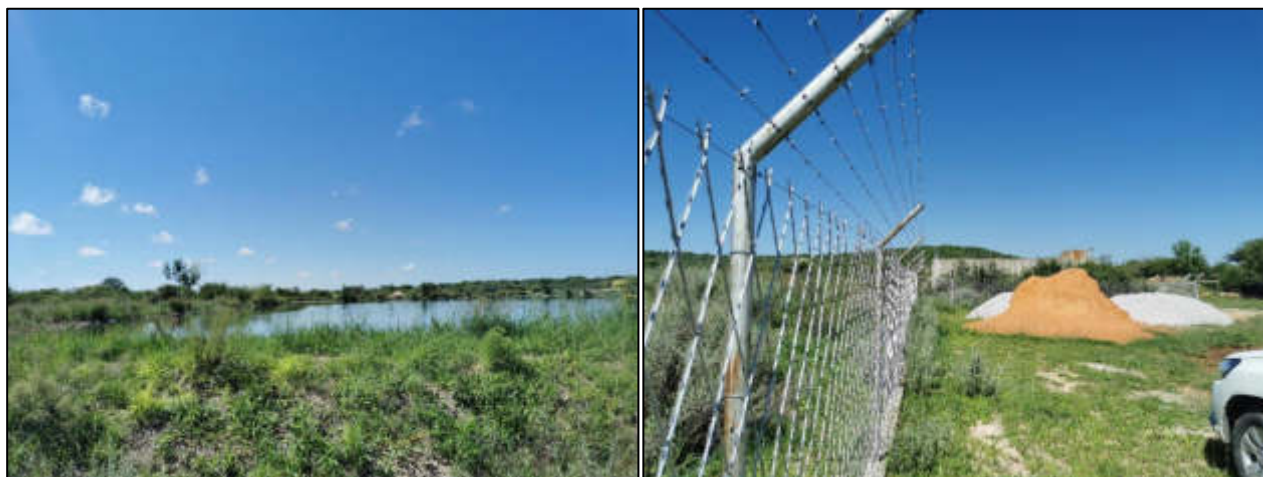
Figure 21: The existing wastewater treatment dam, east of the project site
