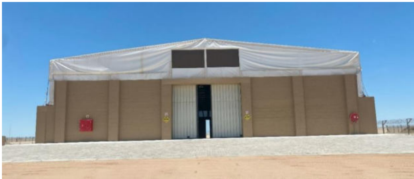
Figure 4: One of the storage facilities.
