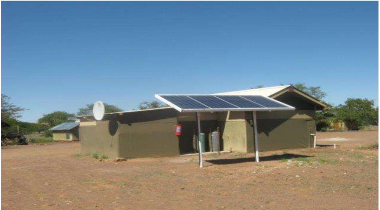
Figure 6: Staff village with solar plant
