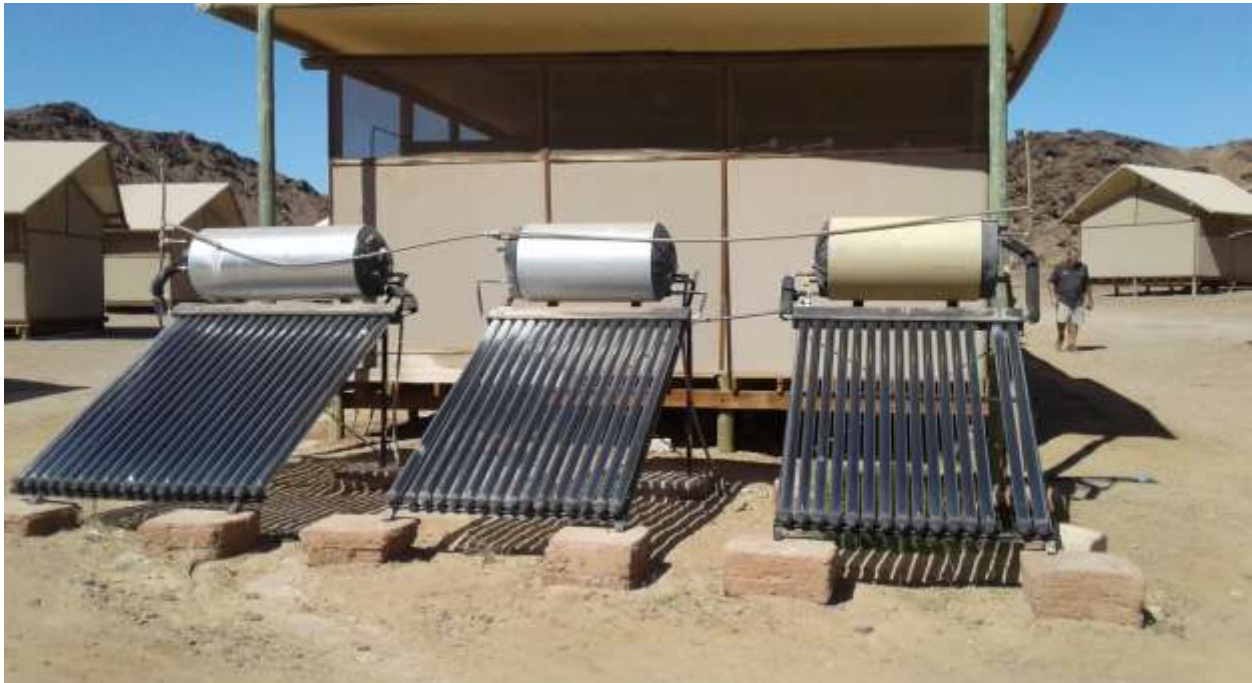
Figure 8: Staff village solar geysers and ablution block
