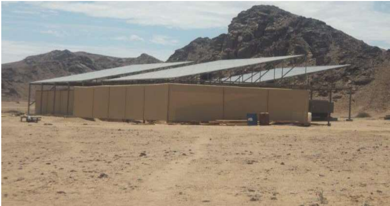
Figure 7: Solar plant and workshop area
