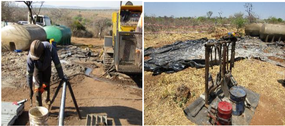
Figure 12 - Drill rig, sumps and water tanks at Drill-hole site: NANAND000019
