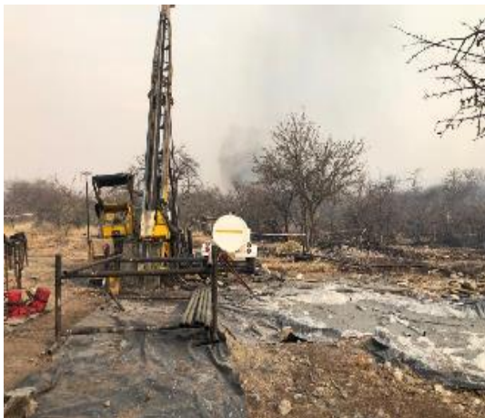
Figure 16 - Drill rig and sumps at site: NANAND000021
