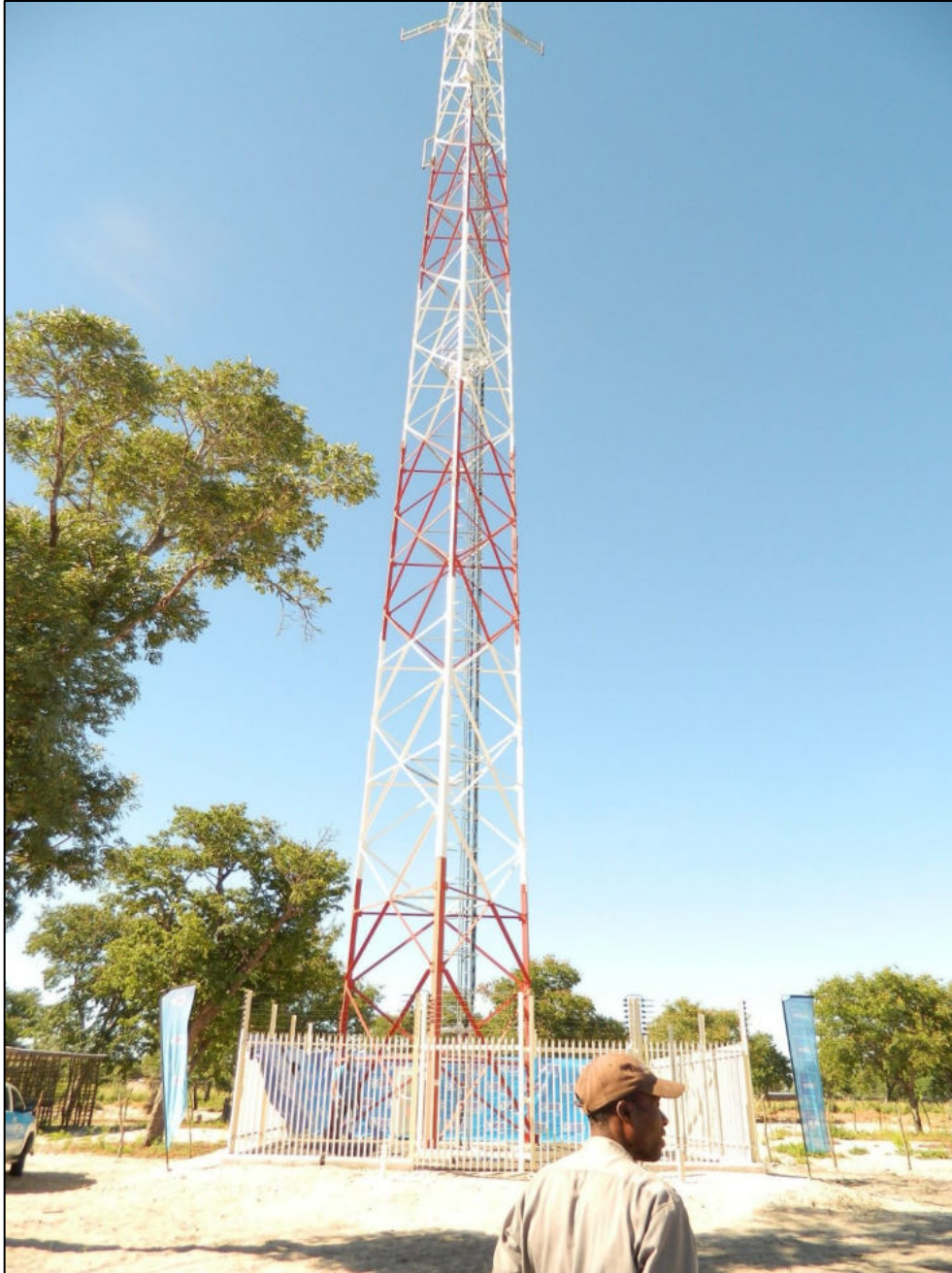
Figure 2: Example of a Freestanding Lattice Telecommunication Tower
