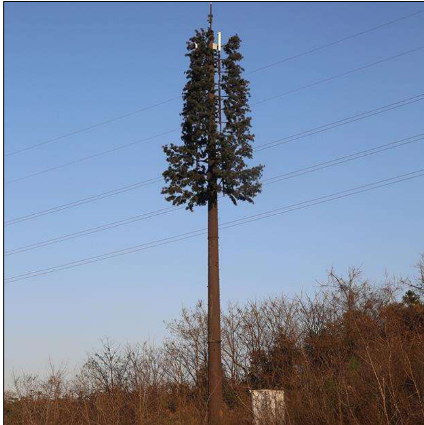
Figure 2: Example of a camouflaged tree telecommunication tower (source: https://www.steeltowerchn.com/camouflaged-tower/camouflage-tower-for-telecom-site/ )
