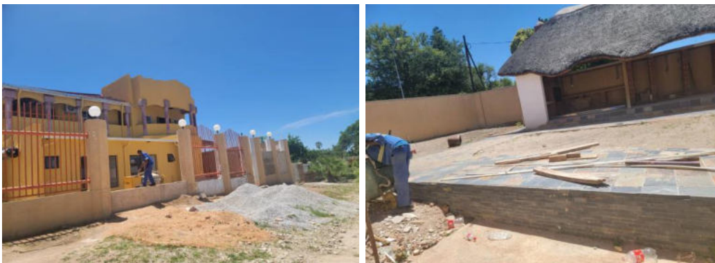
Picture: Structure on erf RE 1064
