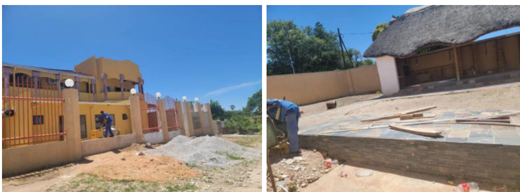
Picture 1: Structure on erf RE 1064
