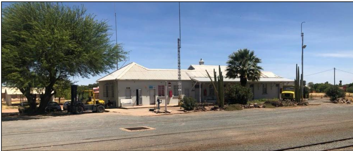
Figure 4: Railway Station buildings
