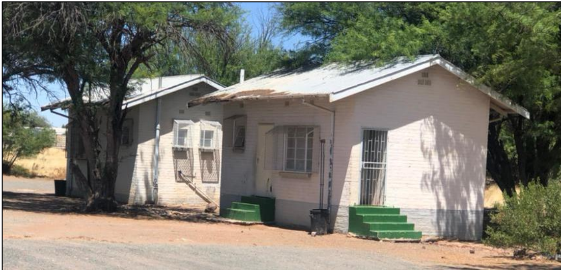
Figure 1: Other buildings observed on site
