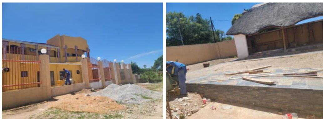
Picture: Structure on erf RE 1064
