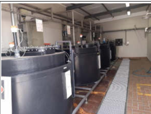
Photo 4-27. Chemical store (inside)
