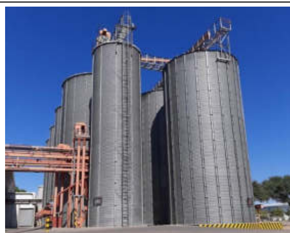
Photo 4-3. Silos for barley storage
