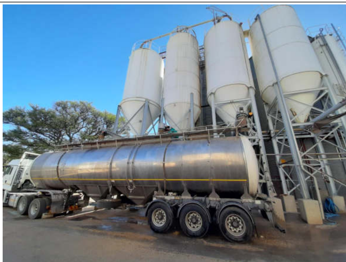
Photo 4-4. Spent malt storage and dispatch
