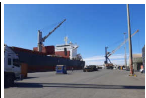
Photo 4-3. View of quay from north to south
