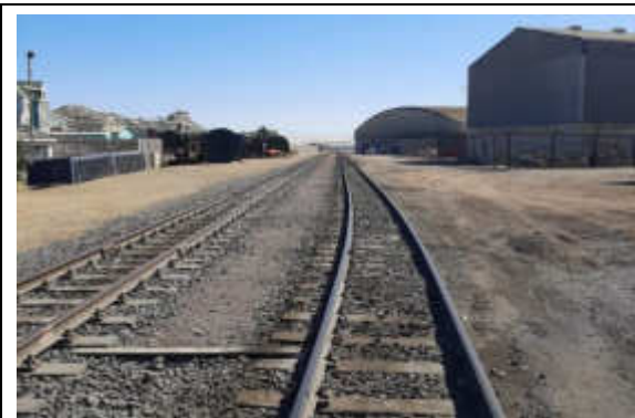
Photo 4-2. Rail siding to future warehouse
