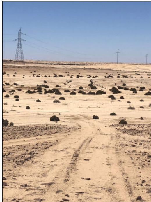
FIGURE 7: PHOTO SHOWING ROADS CROSSING THE POWERLINE CORRIDOR
