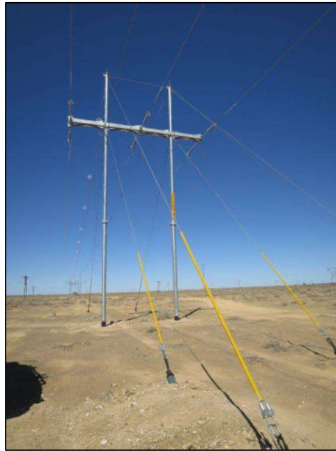
FIGURE 5: PHOTO SHOWING AN EXAMPLE OF THE STEEL CABLE STAYS
