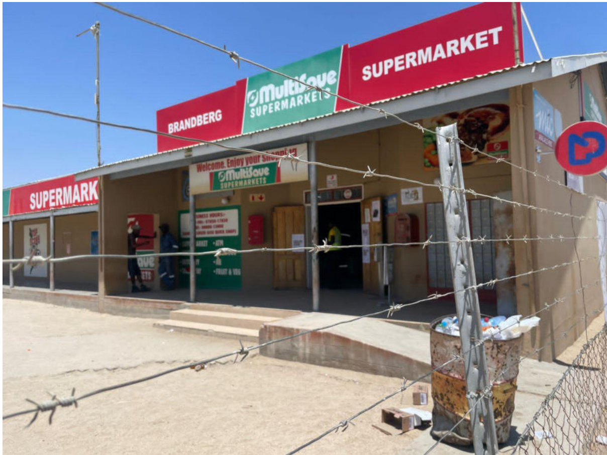
Figure 4: Side View of UIS Multisave Supermarket
