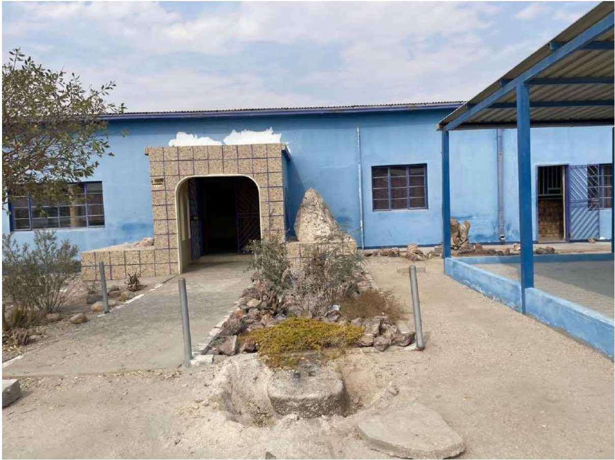
Figure 8: Front View of Okombaye Regional Council
