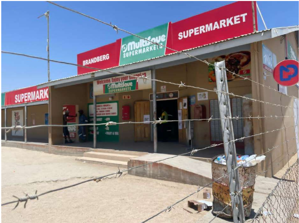
Figure 4: Side View of UIS Multisave Supermarket
