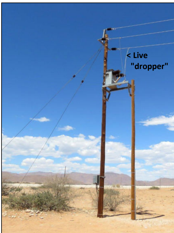
Figure 6 a-b. Examples of typical step-down/transformer installations for the existing 33 kV power line at the customer supply/offtake point at the Solitaire Isolating Station; note the live "dropper", and the stay wires "gapped" by means of an insulator.
