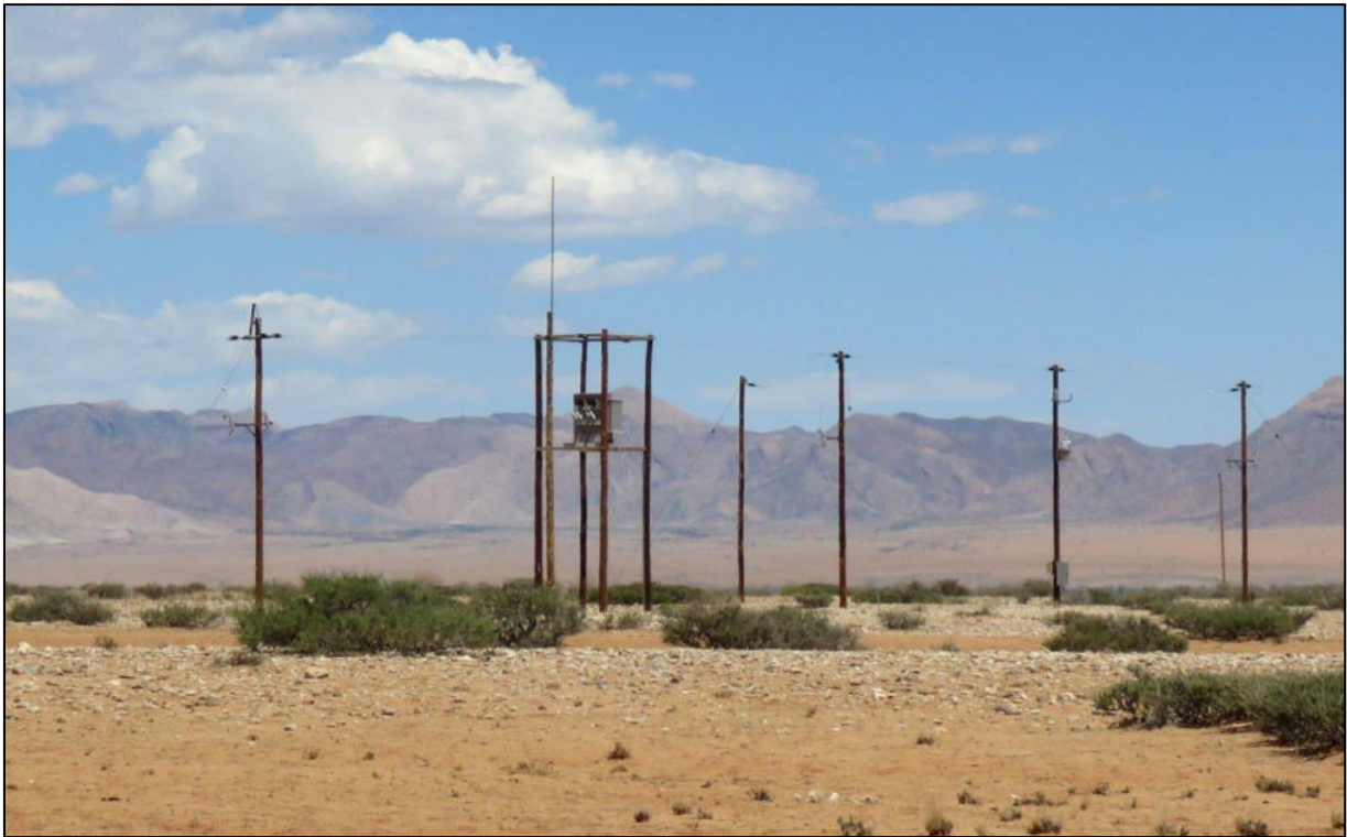
Figure 5. Customer supply / offtake points for the existing 33 kV power line at the Solitaire Isolating Station.
