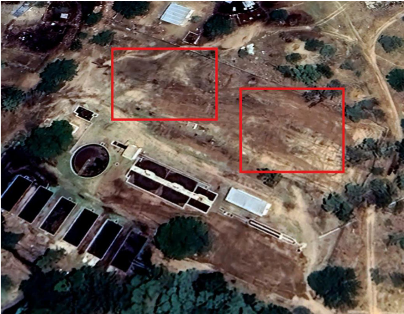
Figure 17 : Okahandja Municipality WWTW Open Area identified for Additional Pond Systems and Sludge Drying
