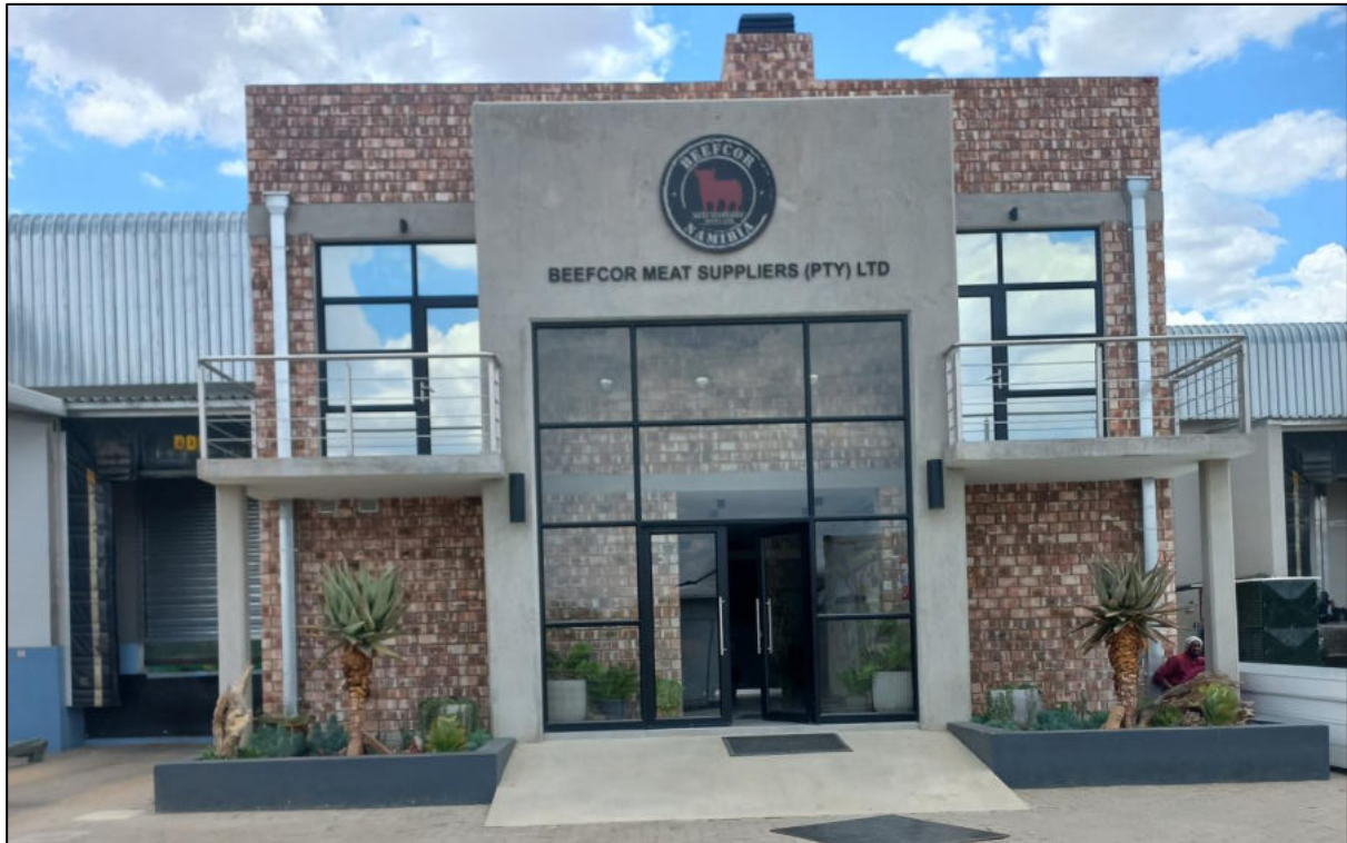
Figure 4: Offices on Beefcor on Project Site
