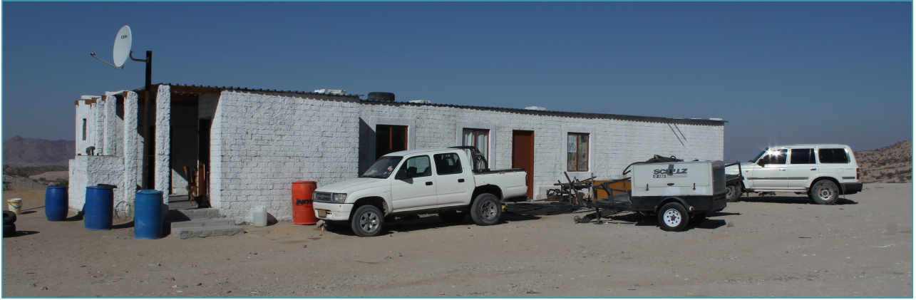
Fig 13: Shows the Staff Accommodation and Current Office Facility (including ablutions), in foreground is the feed collection (light vehicle and compressor equipment)
