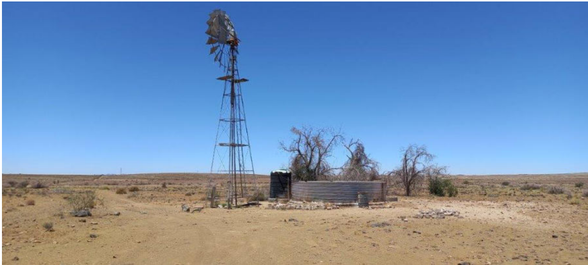
Photo 4.9 – Borehole and Dam that will provide potable water to the Project Site
