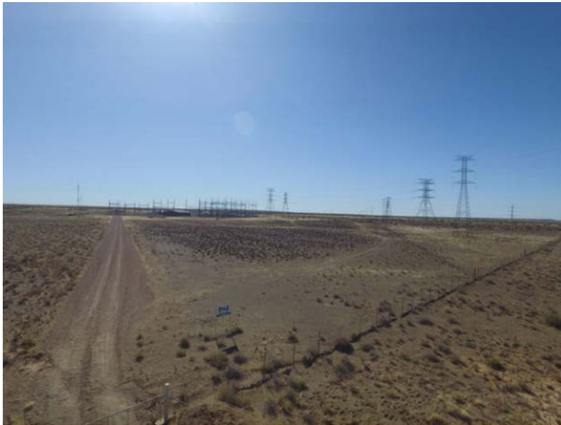
Photo 5.9 – Existing electricity development next to the Project Site
