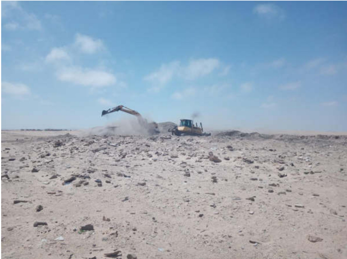
Picture 9 Current land clearing activities on site
