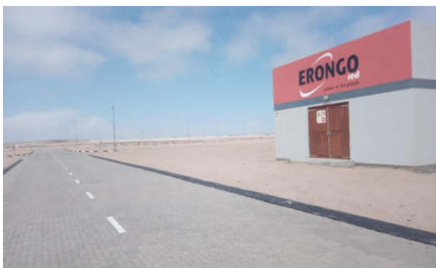
Picture 5 Typical Erongo Red Substation to be constructed on parastatal rezoned portions of POS Erf 231 and 233 after ECC is issued and subdivision and zoning is approved
