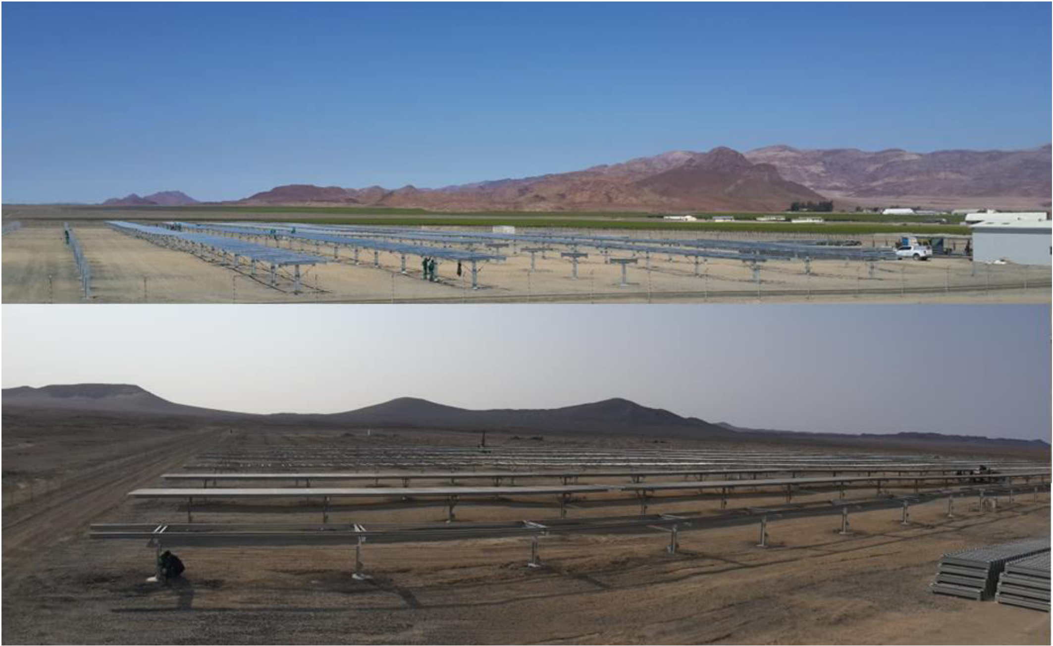
Plate 1.1: The Aussenkehr 5MW Solar PV Park under construction (Source: ALCON, 2019).
