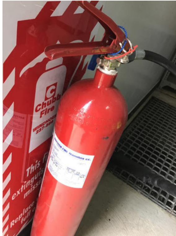
Figure 7 - Valid fire hydrant on site
