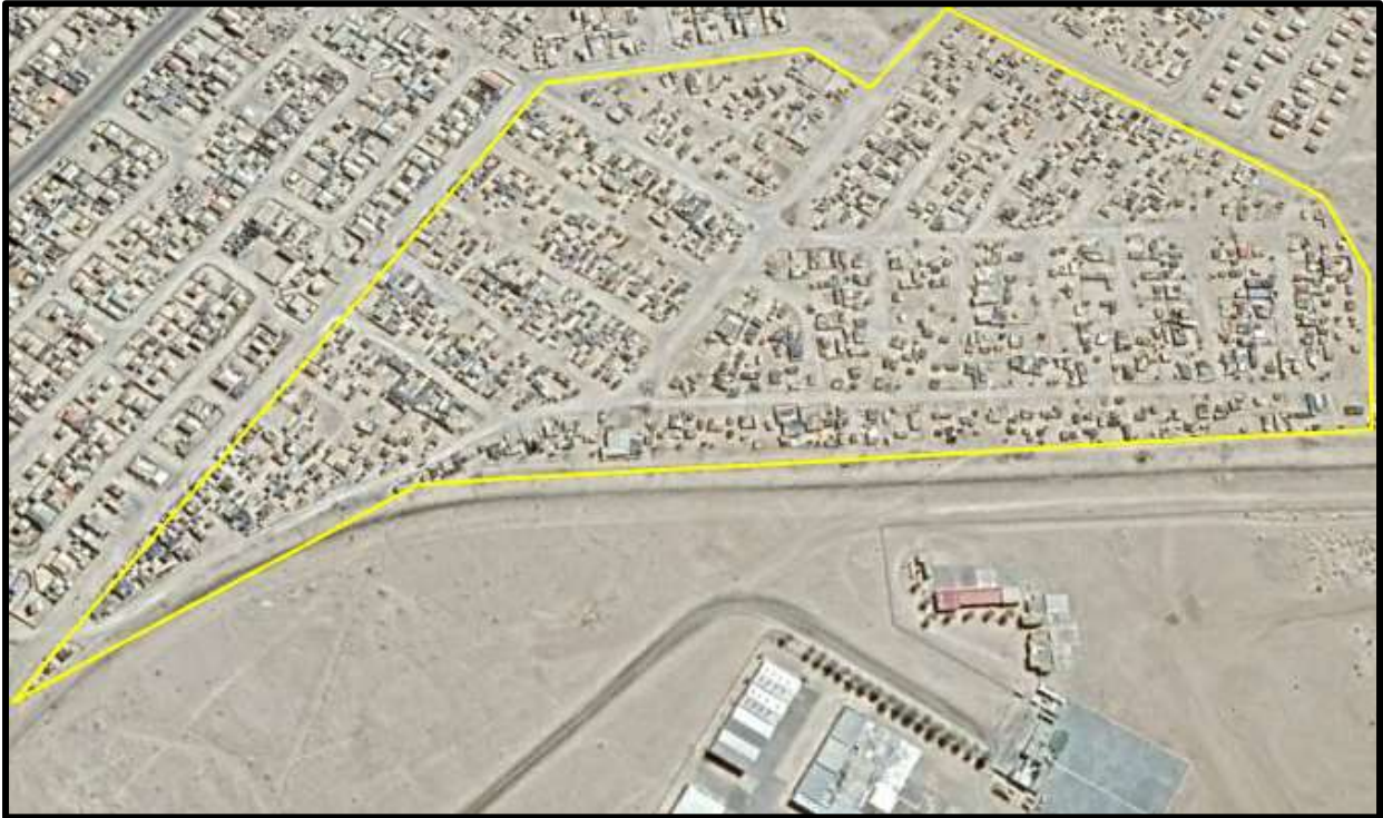
Figure 3: Site overview of Portion 184
