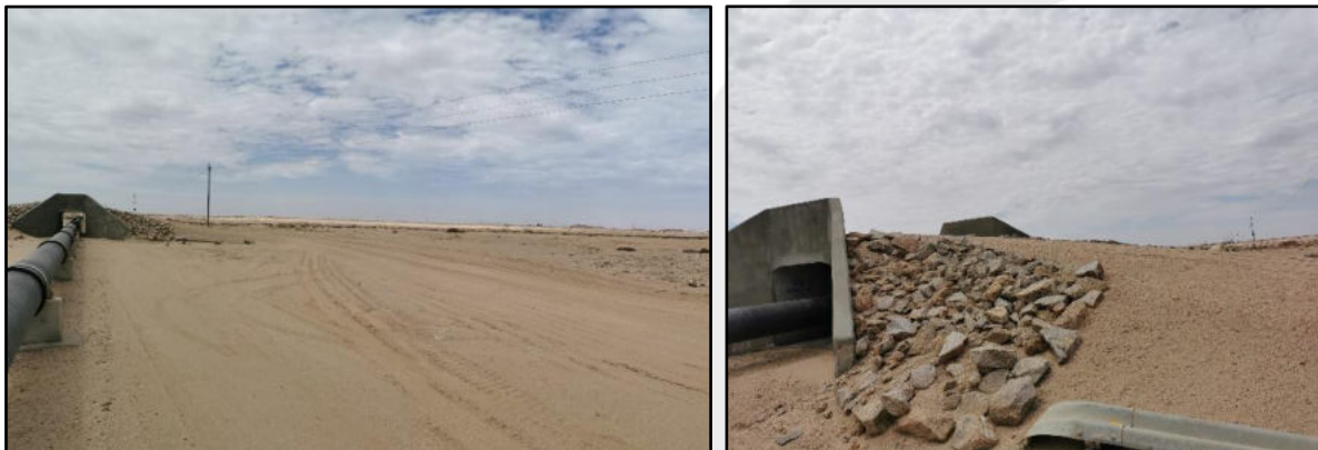
Figure 5.13. The water supply line running the north-eastern side of the Factory
