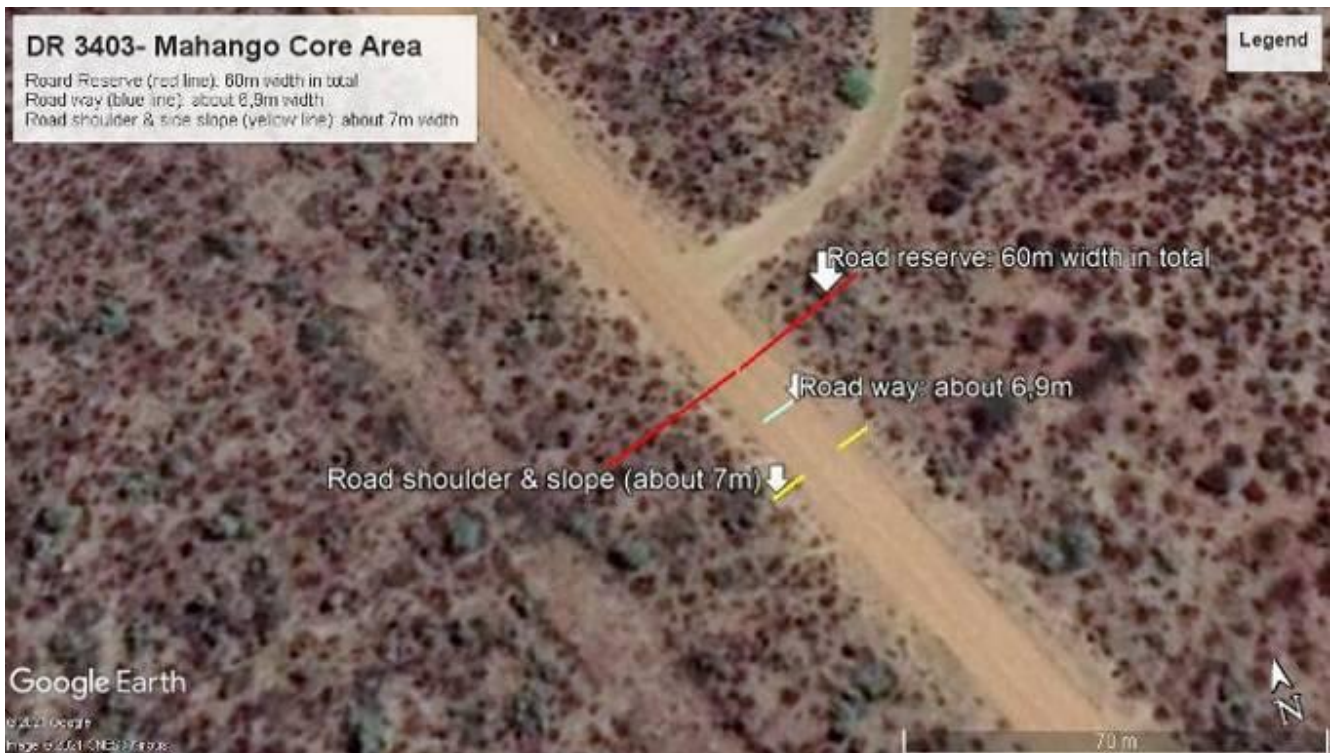
Figure 6: DR3403 Road reserve in Mahango Core Area (Google earth, 2021)
