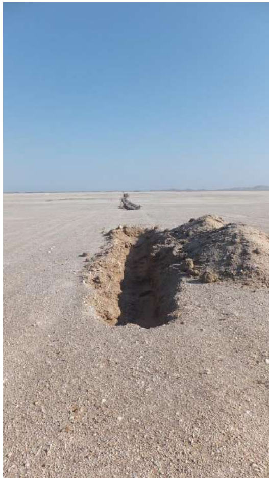
Figure 2: Typical Excavation Pits.
