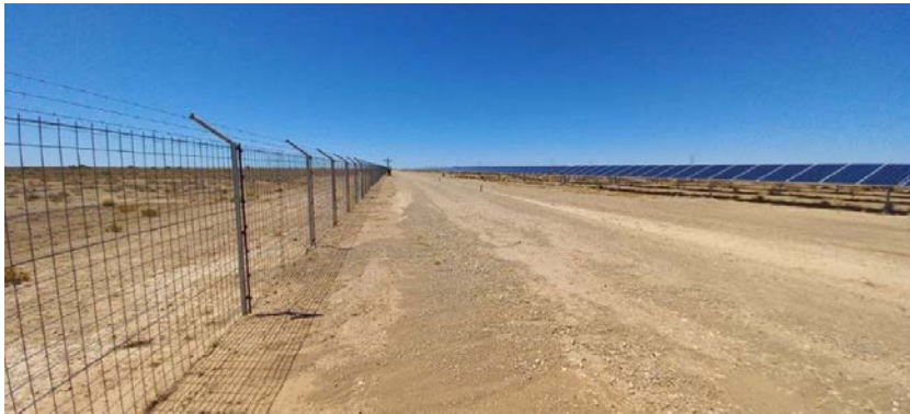
Photo 21 – View of site fence, well maintained and intact.
