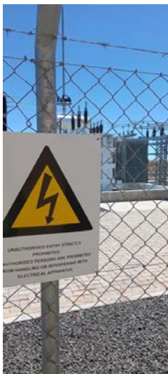
Photo 12 – View of danger sign attached to substation fence.
