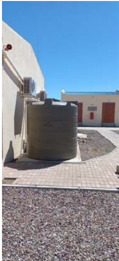
Photo 20 – View of potable water tanks at site office.
