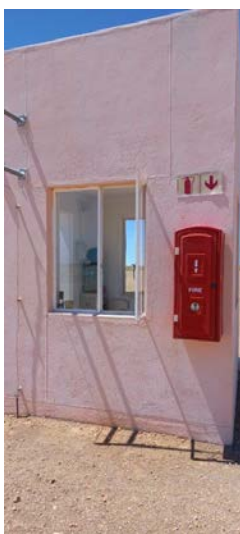
Photo 3 – View of security guard house with fire extinguisher.
