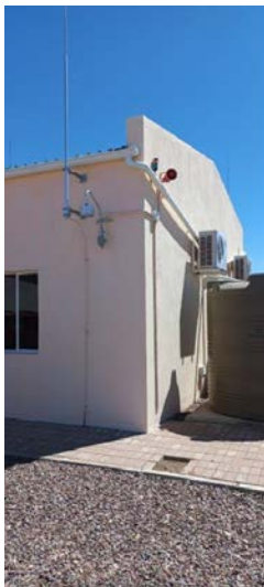
Photo 19 – View of site office with emergency siren.
