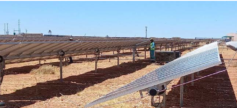
Photo 22 – View of workers doing basic maintenance to PV panels.
