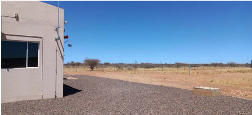
Photo 17 – View of site office with emergency siren.
