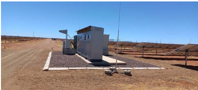
Photo 19 – View of site inverter, well maintained and area surrounding equipment kept clean.
