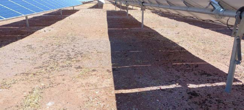
Photo 21 – View of lane in between PV sections have sparse vegetation cover.
