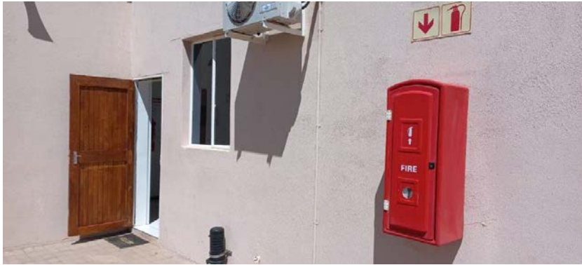
Photo 4 – View of site office with fire extinguisher.
