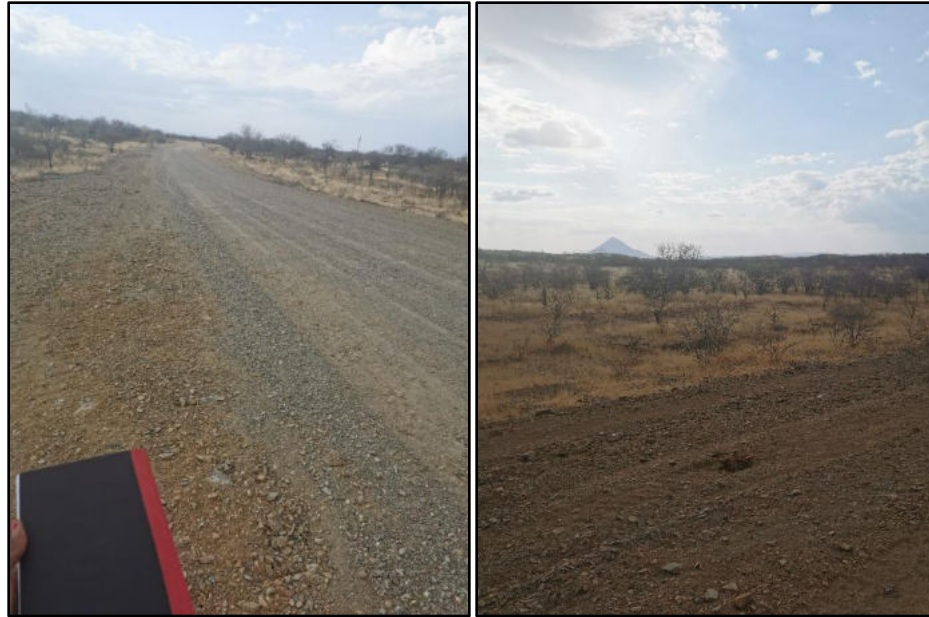
Figure 15: Single track access road from the northern side of the EPL to the south (Omatjete)
