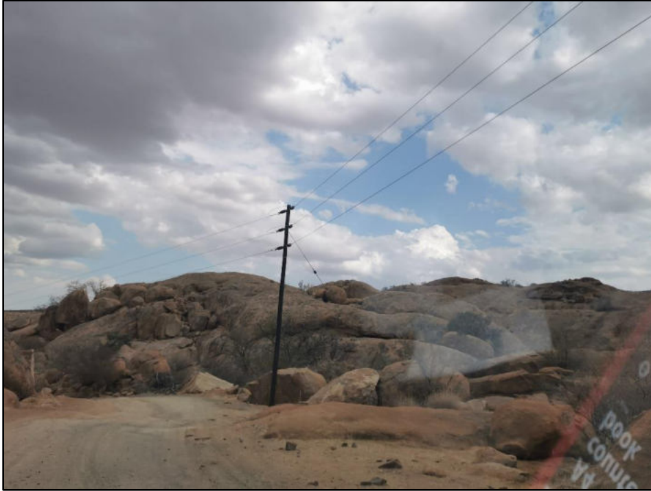
Figure 14: Powerline connecting the existing mining operations to the Okongwe-Otjohorong line
