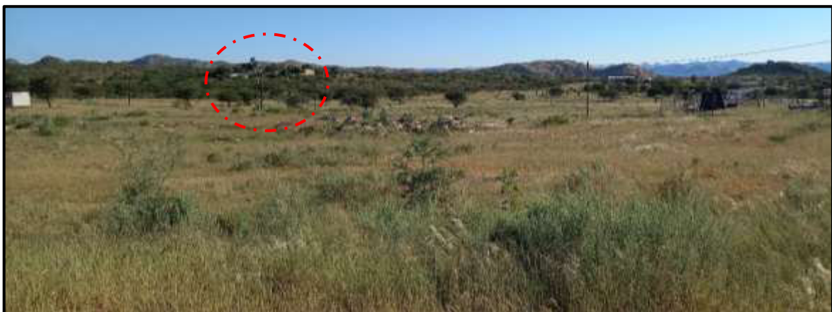
Figure 7: Looking northwest of the property with a Transformer in a Circle
