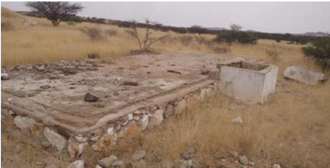
Figure 7; Building remnants (Source: Authors 2022).
