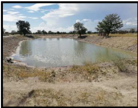
Figure 13: Excavation dam (dugout) on site
