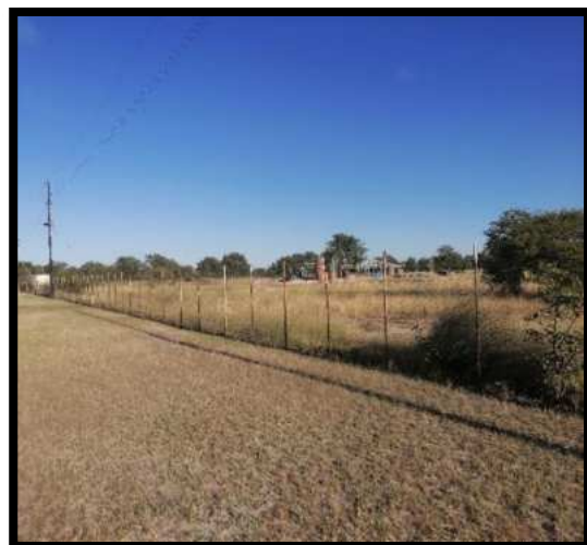
Figure 16: Perimeter fence (rear view)
