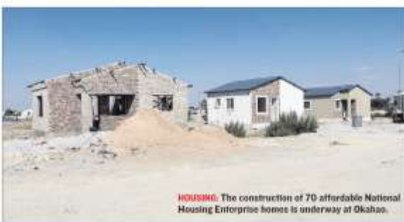
HOUSING: The construction of 70 affordable National Housing Enterprise homes is underway at Okahao.
