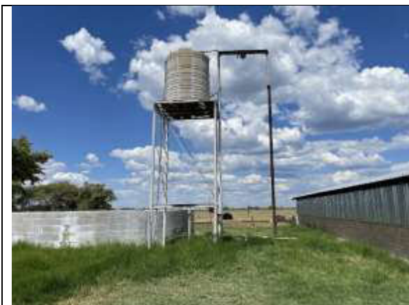
Photo 4-17 Raised water tanks for domestic use
