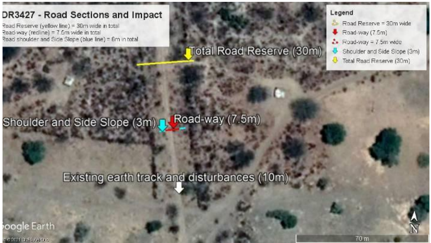
Figure 6: DR3427 Road reserve in a typical land use in the area (Google earth, 2021)
