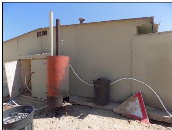
Figure 1-4: Donkey Boiler on site
