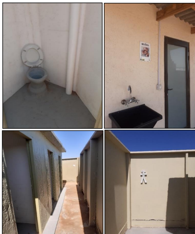
Figure 1-5: ablution facilities available at the camp
