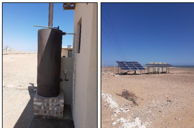
Figure 1-4: Donkey Boiler and Solar panels on site
