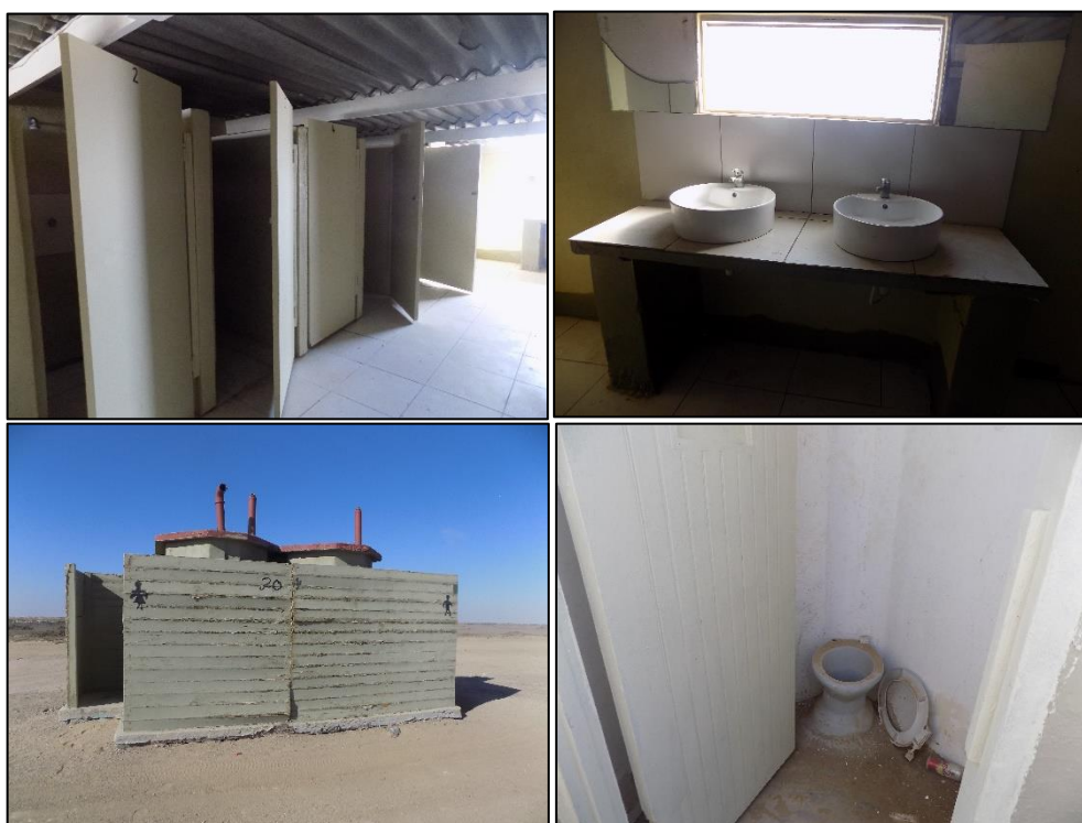
Figure 1-4: Ablution facilities on site
