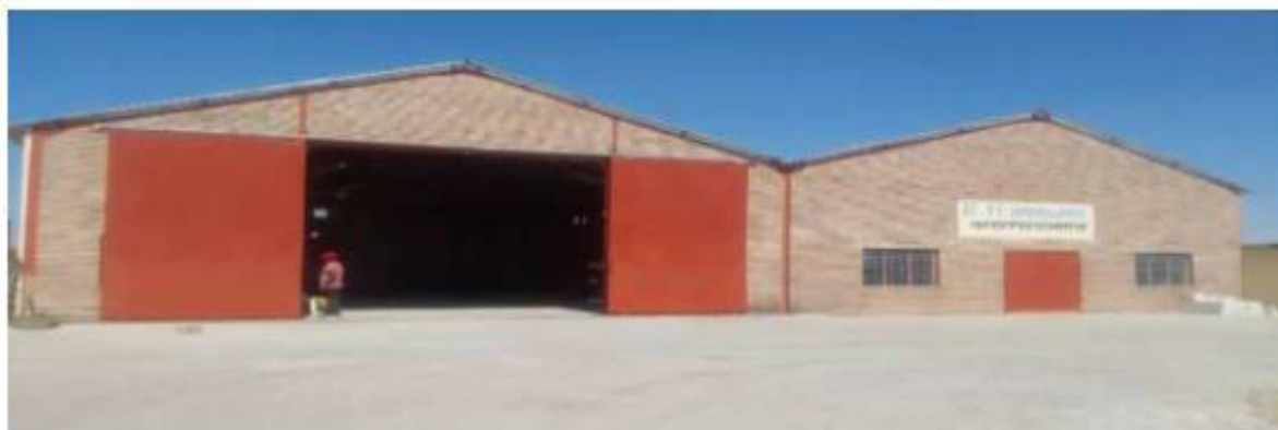
Figure 3: Existing BH Spares warehouse building
