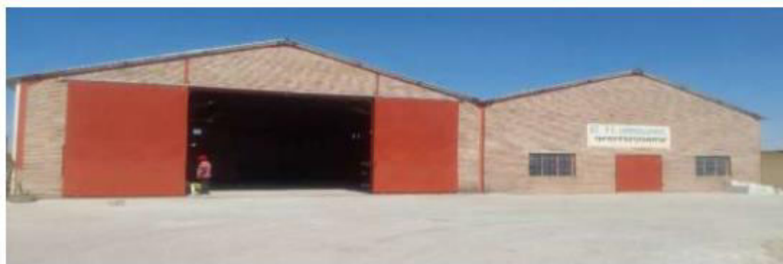
Figure 3: Existing BH Spares warehousing
