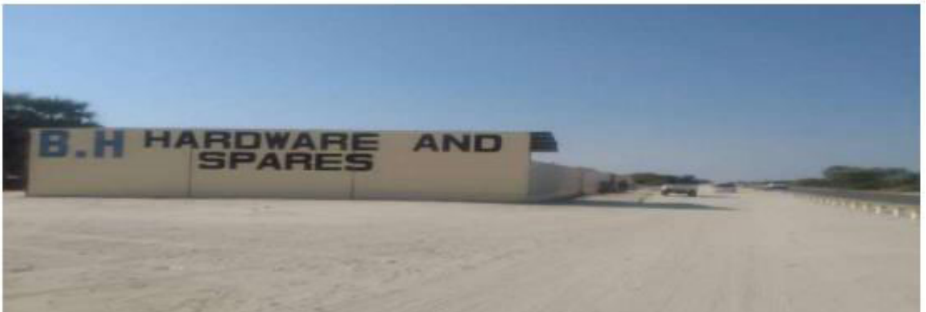
Figure 3: Existing BH Spares warehousing building
