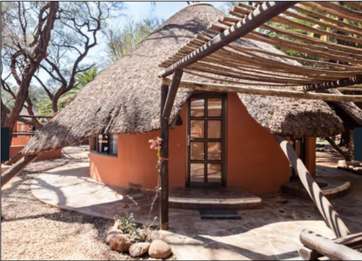
Figure 5: Accommodation facility at Lodge
