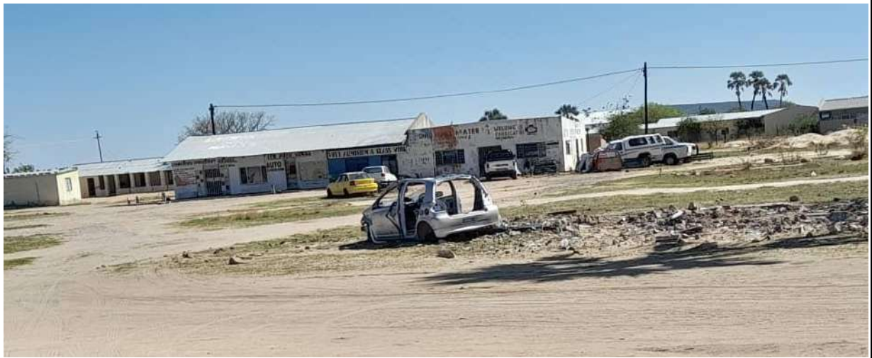
Figure 10: View around the middle of Erf 1206
