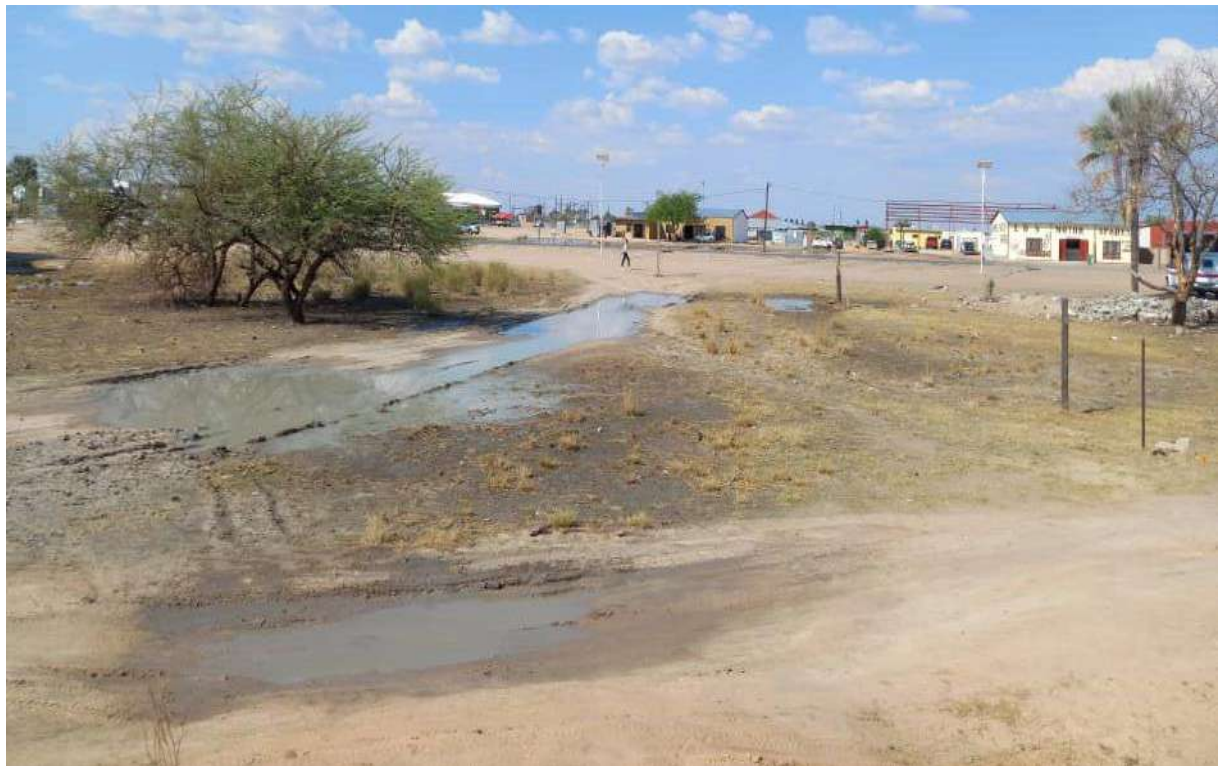
Figure 5: View Looking Eastwards. Note Standing Water and Level of the C46 East of the Site.
