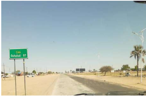
Fig. 11: Standing on C46 Looking South
