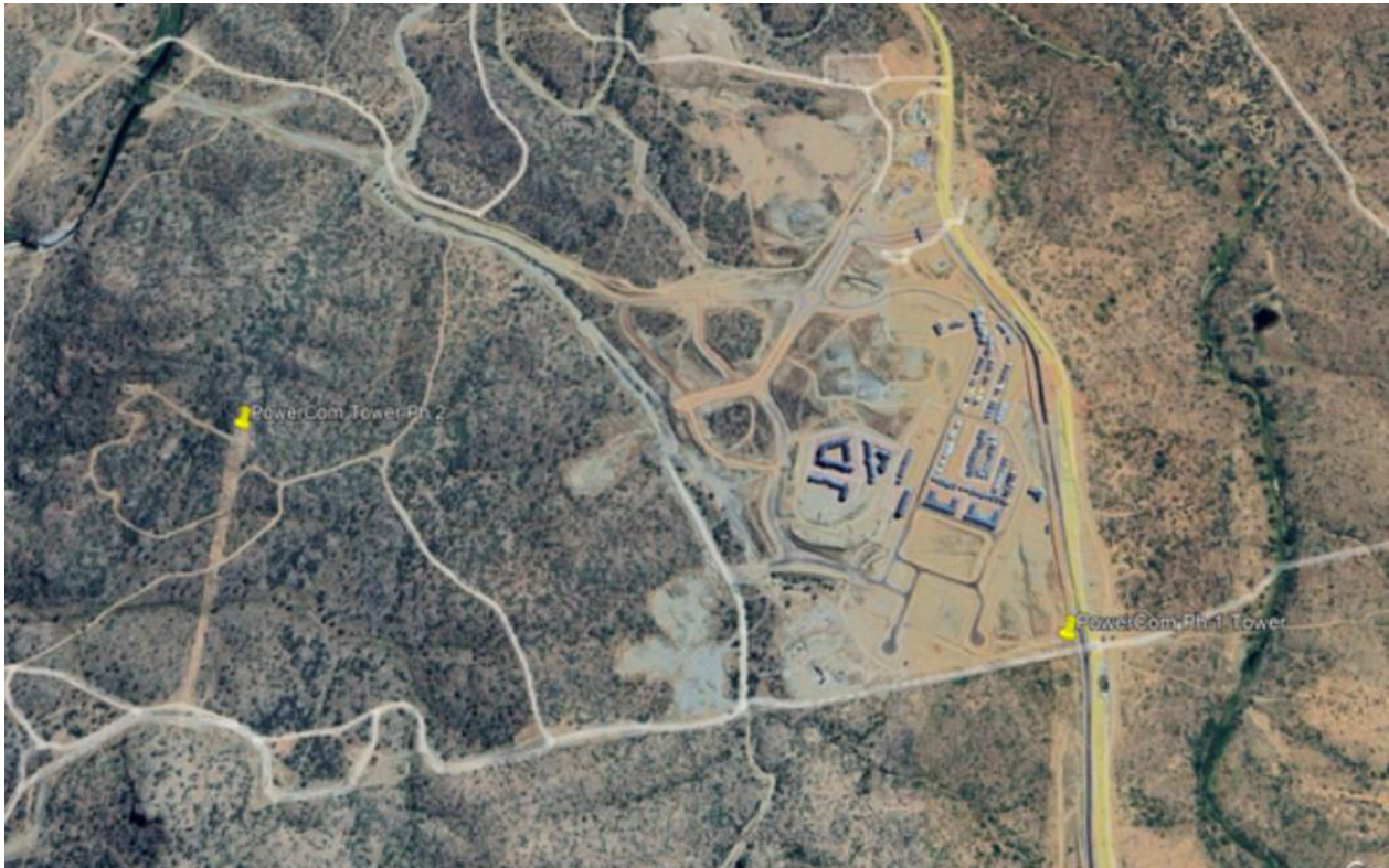
Figure 1: Ongos Portion 8 & 9 Township Telecommunications towers location
