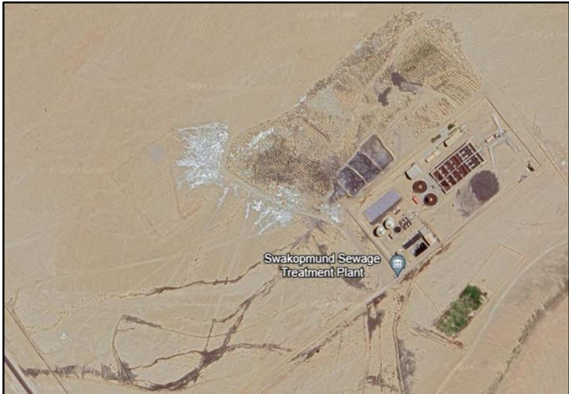
Figure 17 Risk of overflow from the existing STP.
