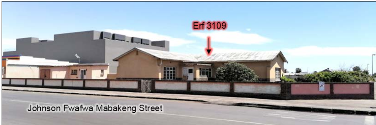
Figure 8: Photo of the former house on Erf 3109 Walvis Bay (Date: 18 Jan 2022).
