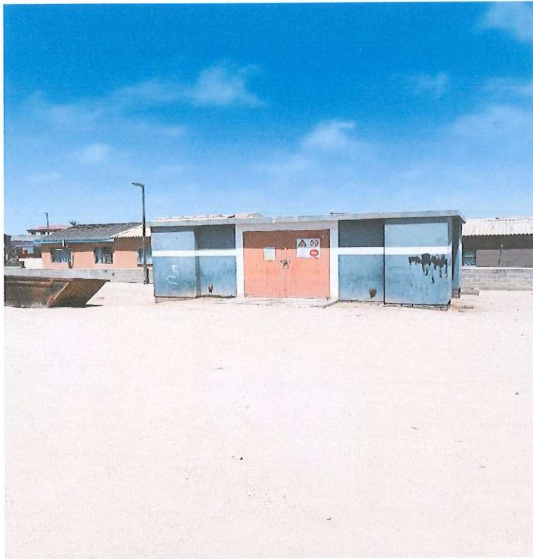
Picture indicates the Electrical Substation of Erf 4378 Mondesa Ext No. 3
